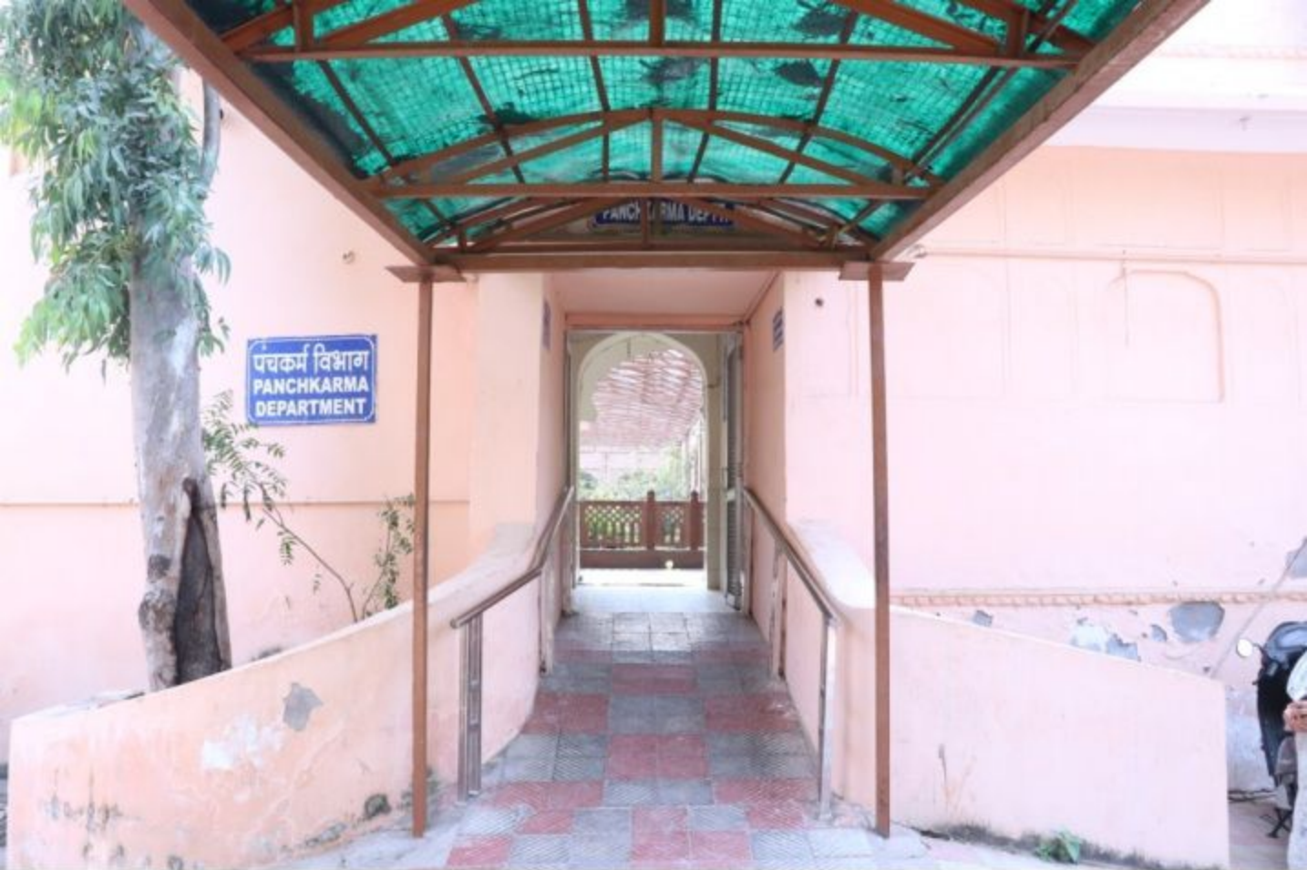
Ramp in Panchkarma Department
